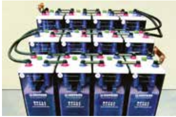
Fig. 5-16: Using row connectors and step connectors
