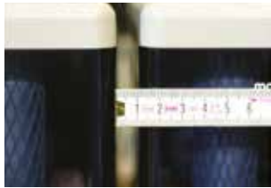
Fig. 5-13: 10 mm clearance between the batteries
