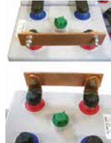
Fig. 5-18: Installing the end terminals (connection plates)
